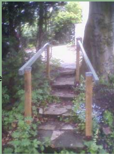
Handrails on steps to butterfly & bee garden
